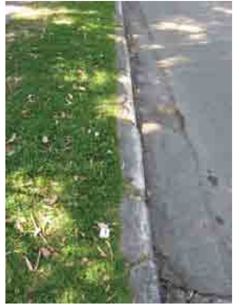
Figure 3-2 Sandstone kerb in Reserve Road, adjacent to Precinct 1 - Core Hospital Precinct
