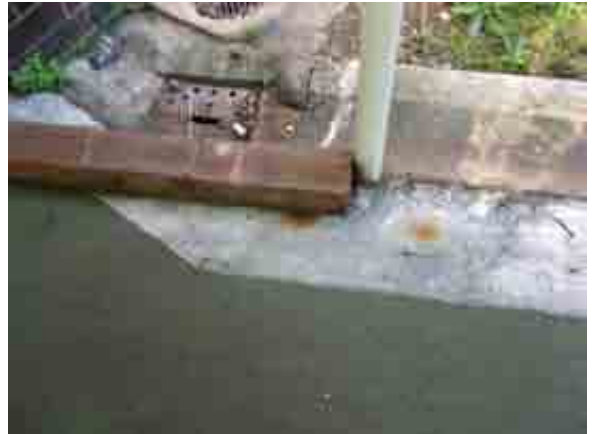
Figure 3-6 A combination of brick and concrete kerbing, east of Building 32
