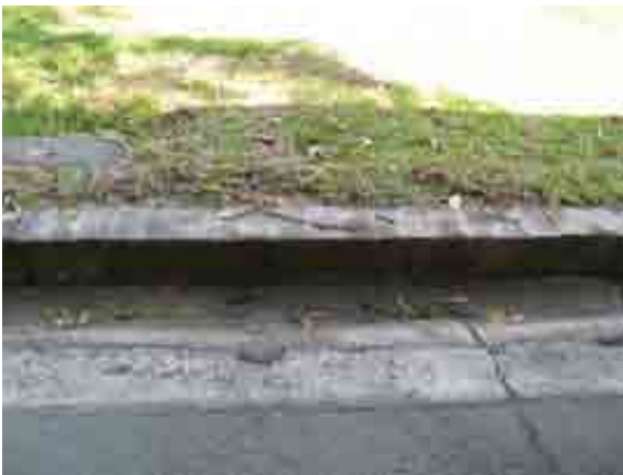
Figure 3-17 Kerb and guttering constructed of brick and concrete, west of Building 19
