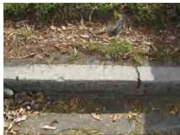
Figure 3-24 Concrete kerb and gutter in the vicinity of Building 22
