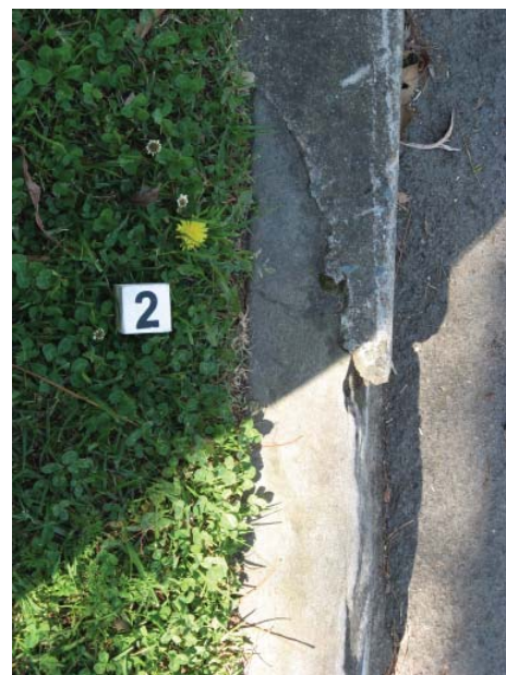
Figure 3-26 Sandstone kerbing, partially covered with concrete, in Reserve Road, adjacent to Precinct 6 - UTS Precinct
