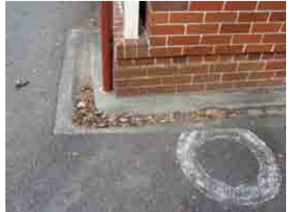
Figure 3-16 Concrete drain at the north west corner of Building 17
