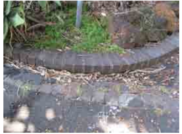
Figure 3-18 Brick kerb and guttering, north east of Building 28
