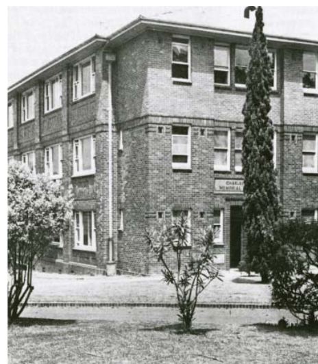
Figure 2-5 Circa 1948 photograph of the Kolling Institute (Building 25)
