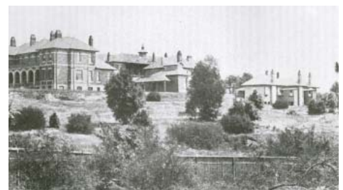
Figure 2-2 1908 view of the Hospital site
