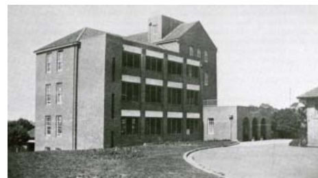
Figure 2-4 Photograph of the Princess Elizabeth Pavilion (Building 35), which was opened in 1934
