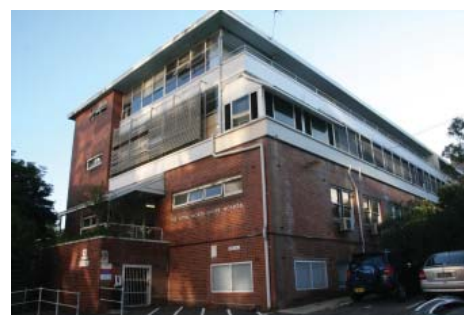
Figure 4-12 Building 10, viewed from Herbert Street
