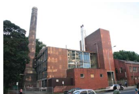
Figure 4-11 Boiler House (Building 21) and chimney, viewed from Herbert Street
