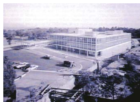
Figure 2-6 Circa 1964 photograph of the Main Block (Building 1)
