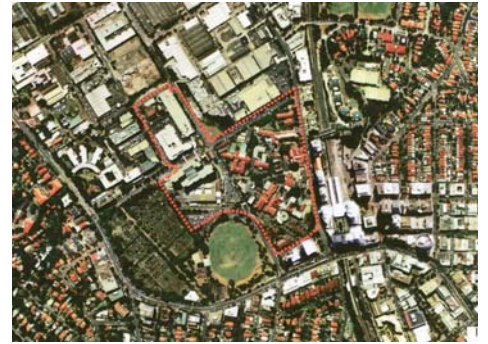
Figure 1-1 Aerial photograph with the Royal North Shore Hospital site boundaries marked in red.
