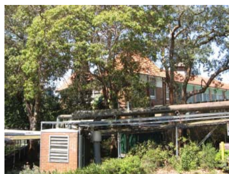
Figure 4-6 North east corner of Building 29
