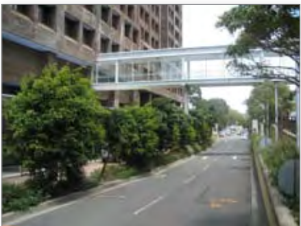
Pedestrian overpass Westbourne Street
