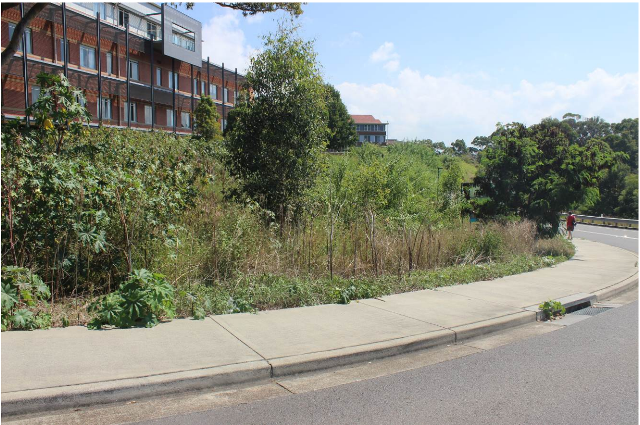
Photograph 8 – Concrete Footpath – Jacaranda Drive
