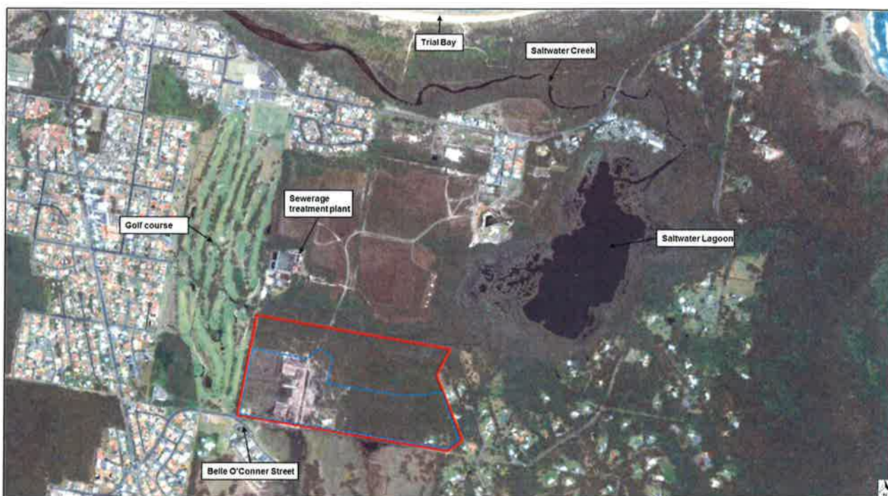
Figure 2: Aerial view of the site location (outlined in red), its surroundings and the subdivision boundary (outlined in blue dashed line) (Base source: Nearmap)
