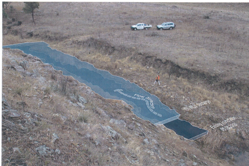
Figure 5.1: A representative model of maximum pipeline flow and an inundation event recorded on 5 August 2008 overlaid on a section of Burra Creek approximately 3.1 kilometres from the preferred project discharge point.
