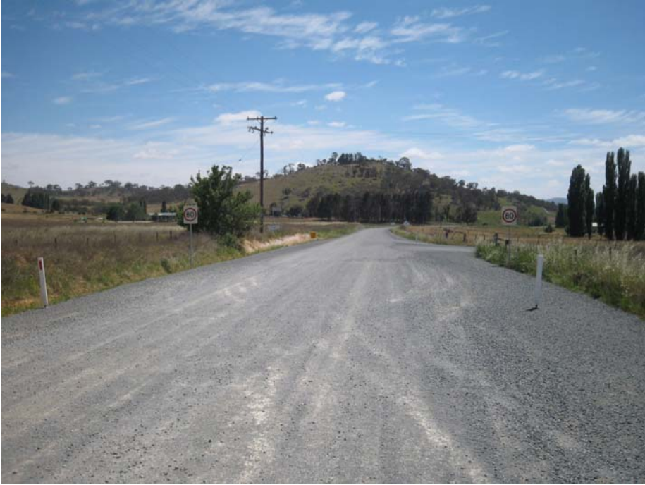
Photo 11: Williamsdale Road at Badgery Road intersection
