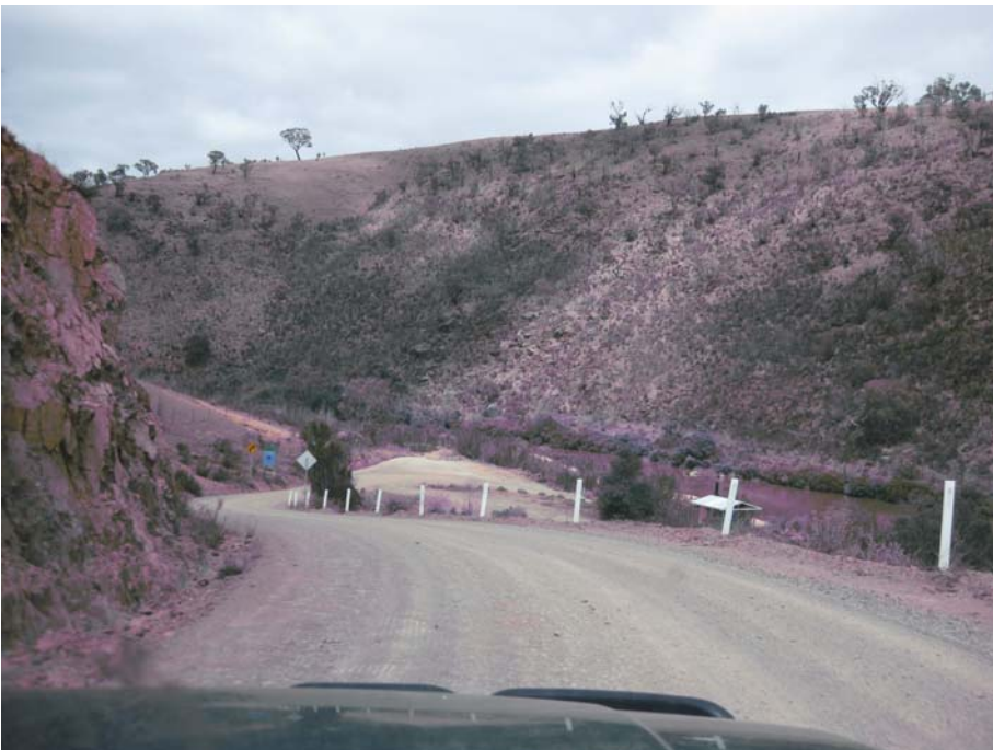
Photo 2: Angle Crossing Road approaching Causeway
