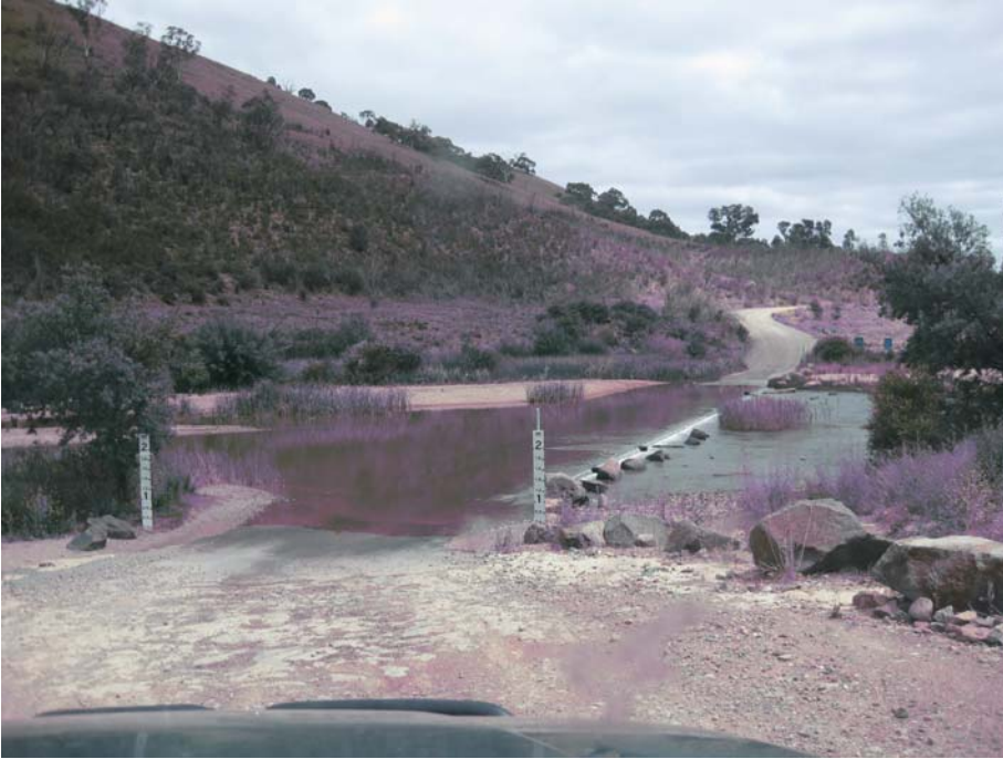
Photo 1: Angle Crossing Road at Causeway
