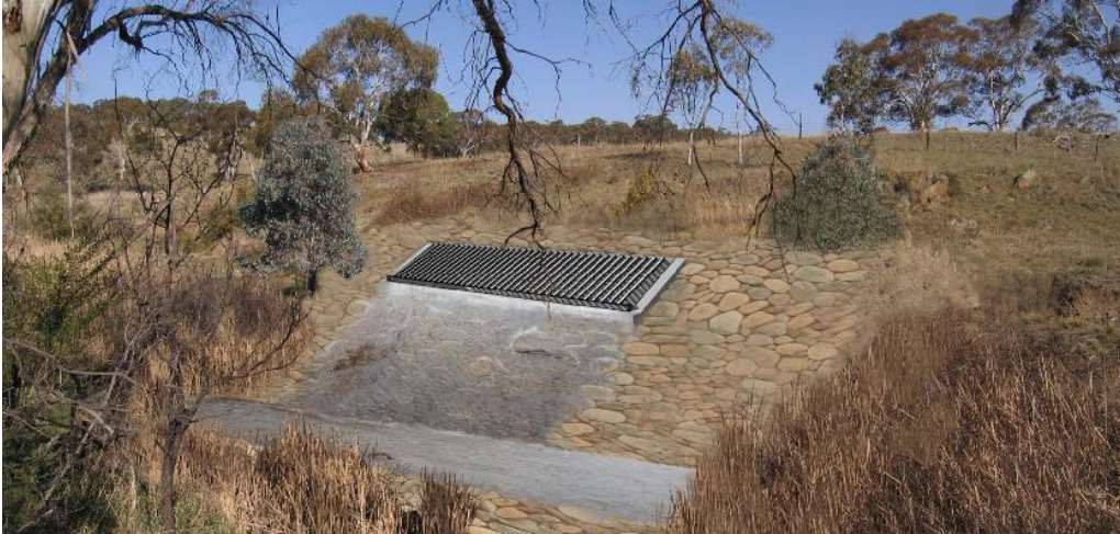
Figure 4.8 Graphical representation of discharge structure
