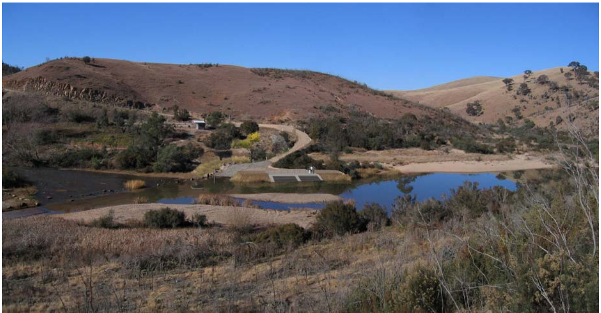
Simulation 1 – Simulation indicating view south west of the intake structure from the north side of the MRC, adjacent to Angle Crossing.
