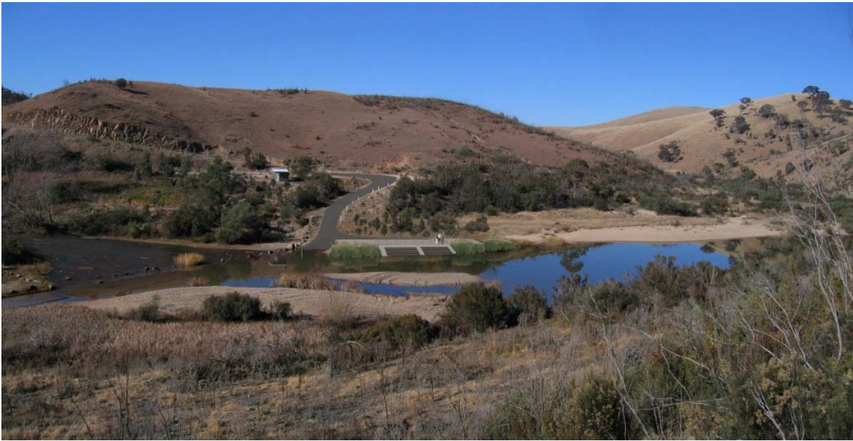
Figure 2.2 Visual representation of intake structure of Angle Crossing
