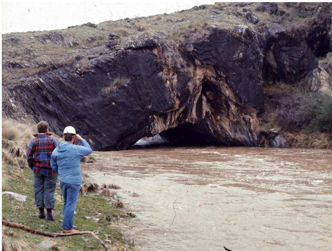
Figure 13. Downstream side of London Bridge during the falling limb of a flood in November 1976
