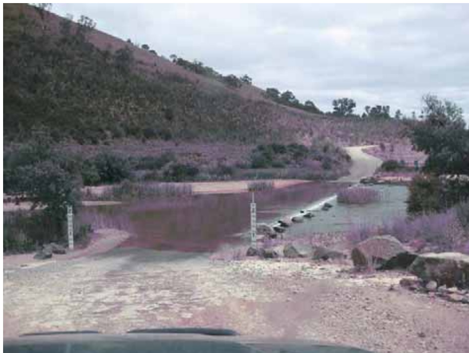
Photo 1: Angle Crossing Road at Causeway
