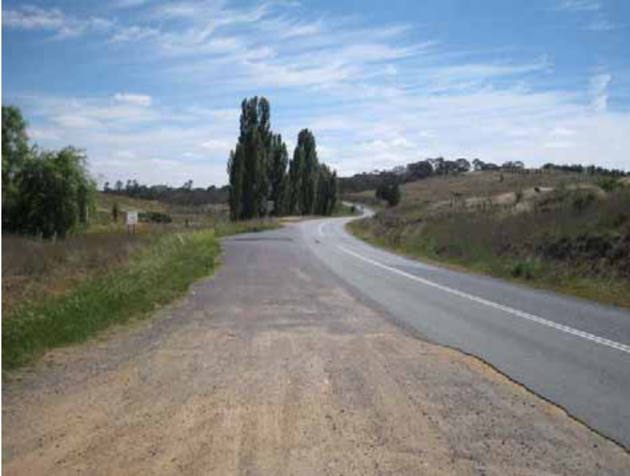
Photo 15: Burra Road northbound approaching Williamsdale Road intersection
