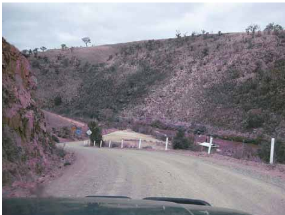
Photo 2: Angle Crossing Road approaching Causeway
