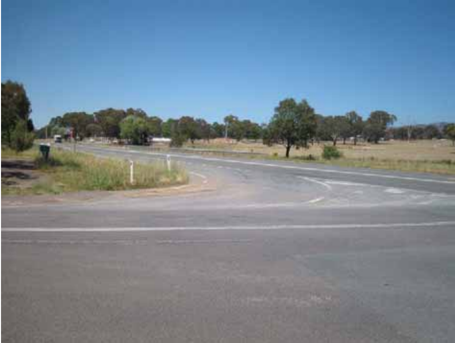
Photo 7: Williamsdale/ Monaro Highway intersection looking south
