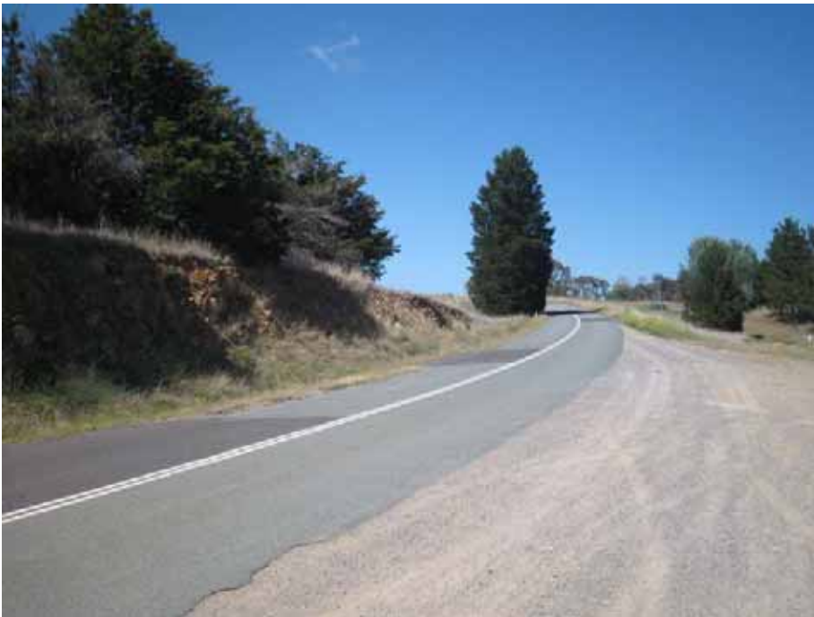
Photo 16: Burra Road southbound from Williamsdale Road
