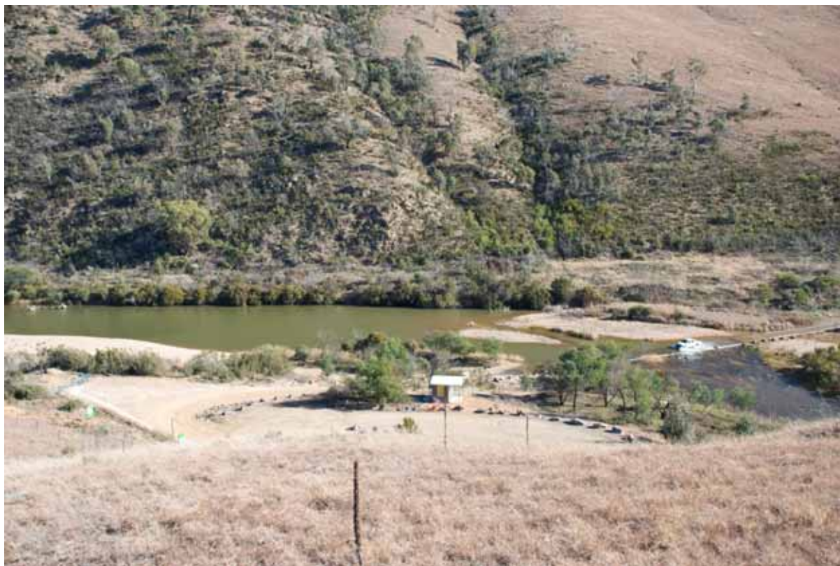
Figure 3.3 Looking west towards Angle Crossing and the intake/low lift pump station site, from the high lift pump station site
