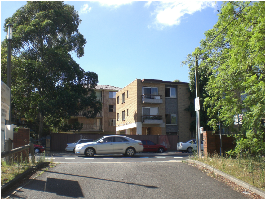
Figure 4 Development across Hawkesbury Road
