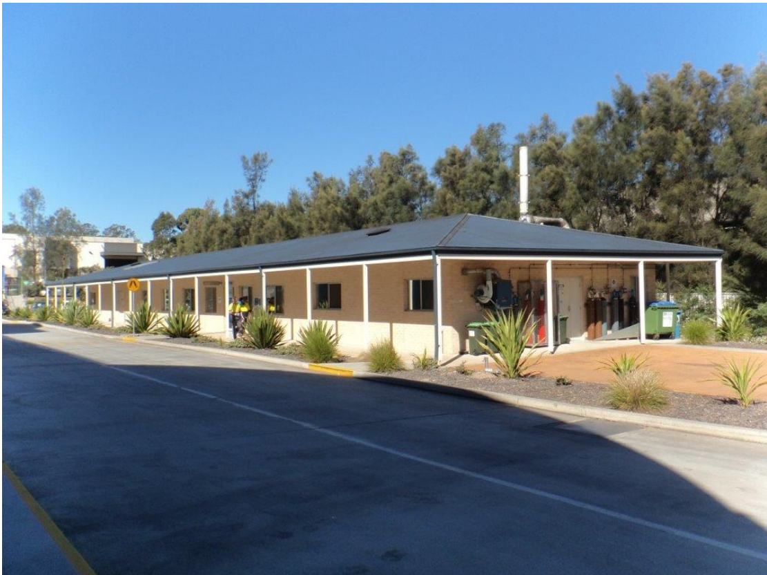
View of the office expansion site looking south-east
