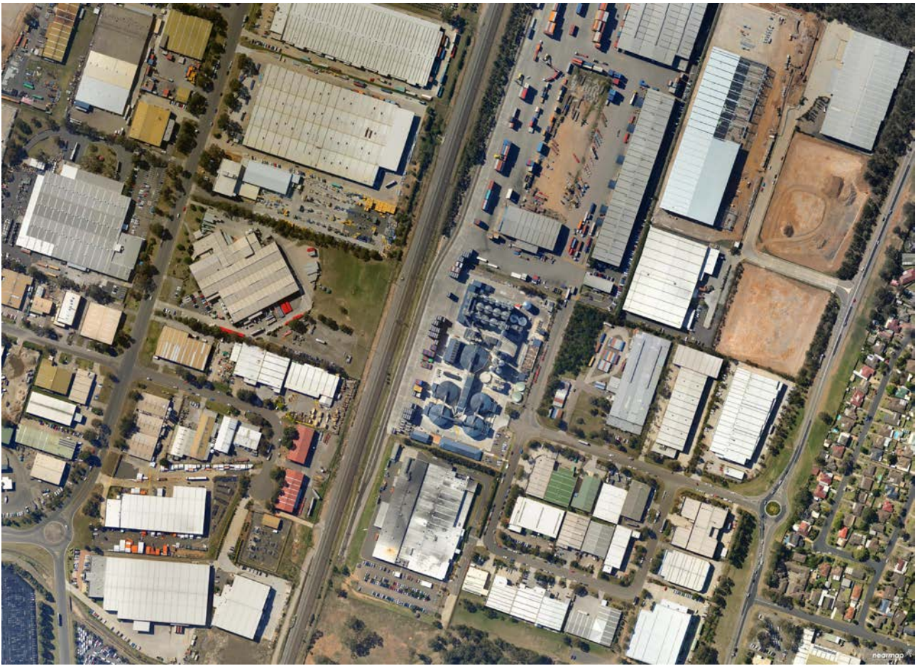
Figure 2: Site in context of surrounding industrial area Source: NearMap
