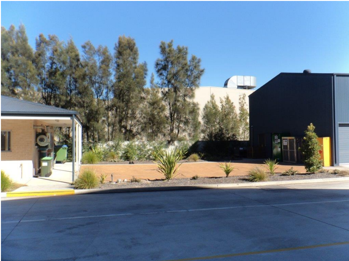
View of the office expansion site looking south
