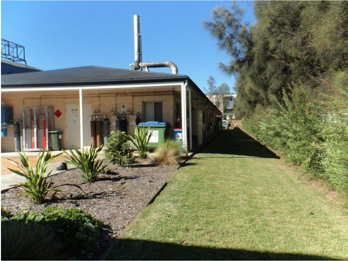
View of the office expansion site looking east
