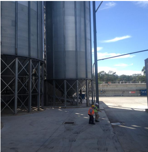
Figure 2-6 Site of two new silos in front of MCC3
