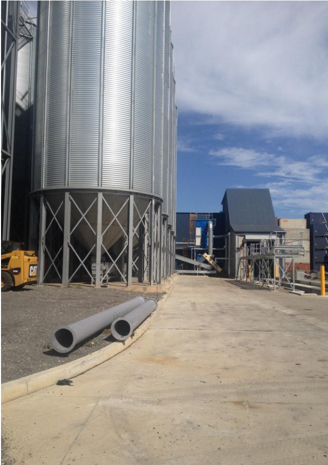
Figure 2-4 Site of proposed eastern most silos adjacent to existing matching silos
