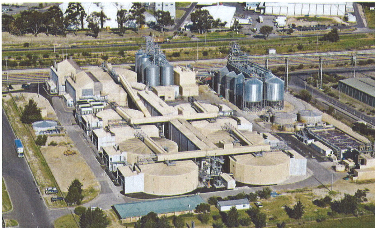
Figure 5: Aerial photograph of existing plant in Forrestfield WA (source: Cardno EA page 35)
