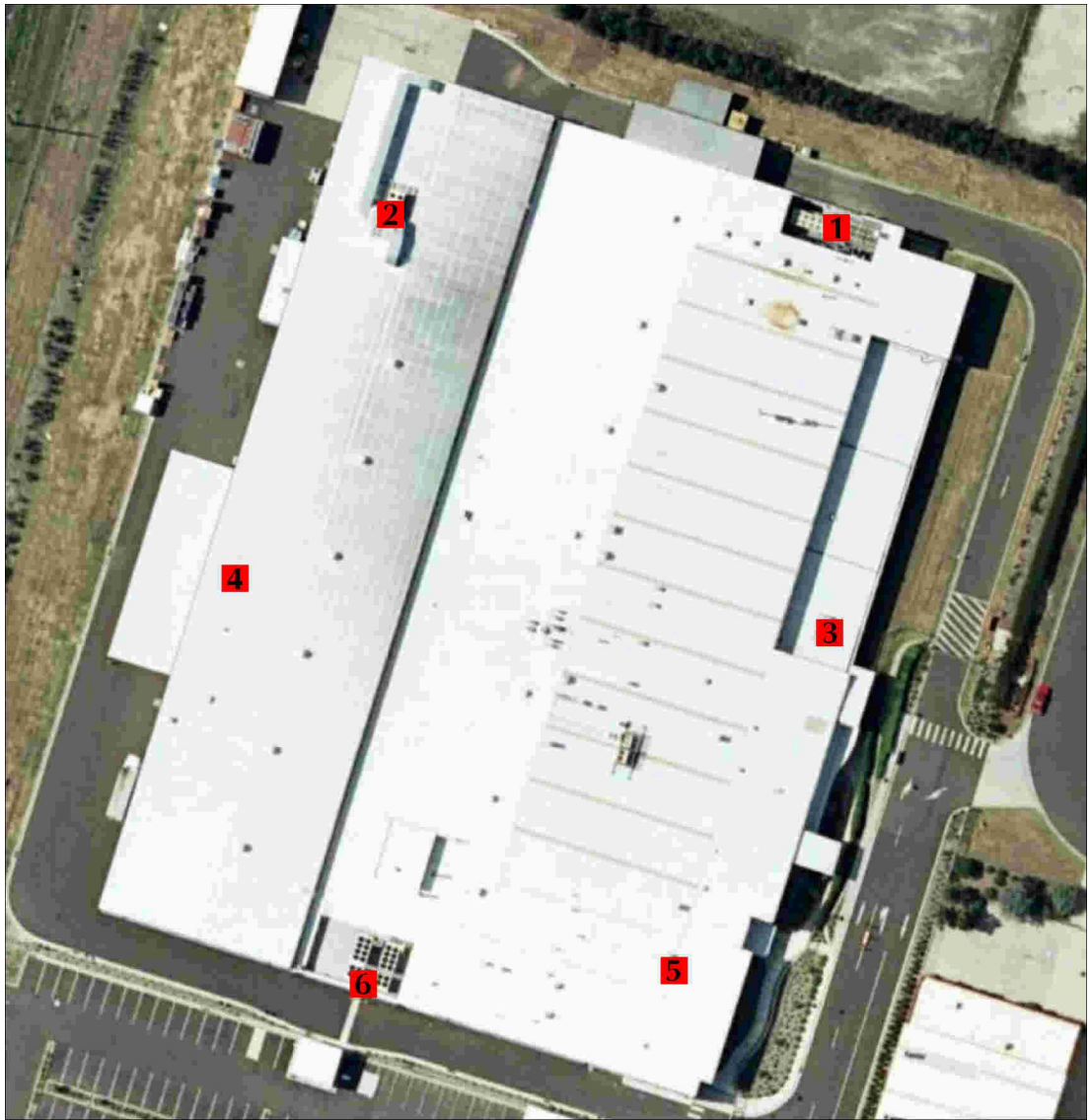
Figure 3: Air-intake points at Lipa Pharmaceuticals
