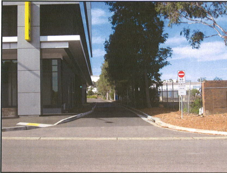
Figure 14 – Rear lane access
