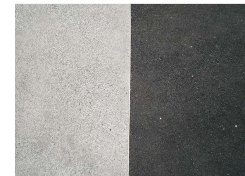
Asphalt paving to the building line AC10.
