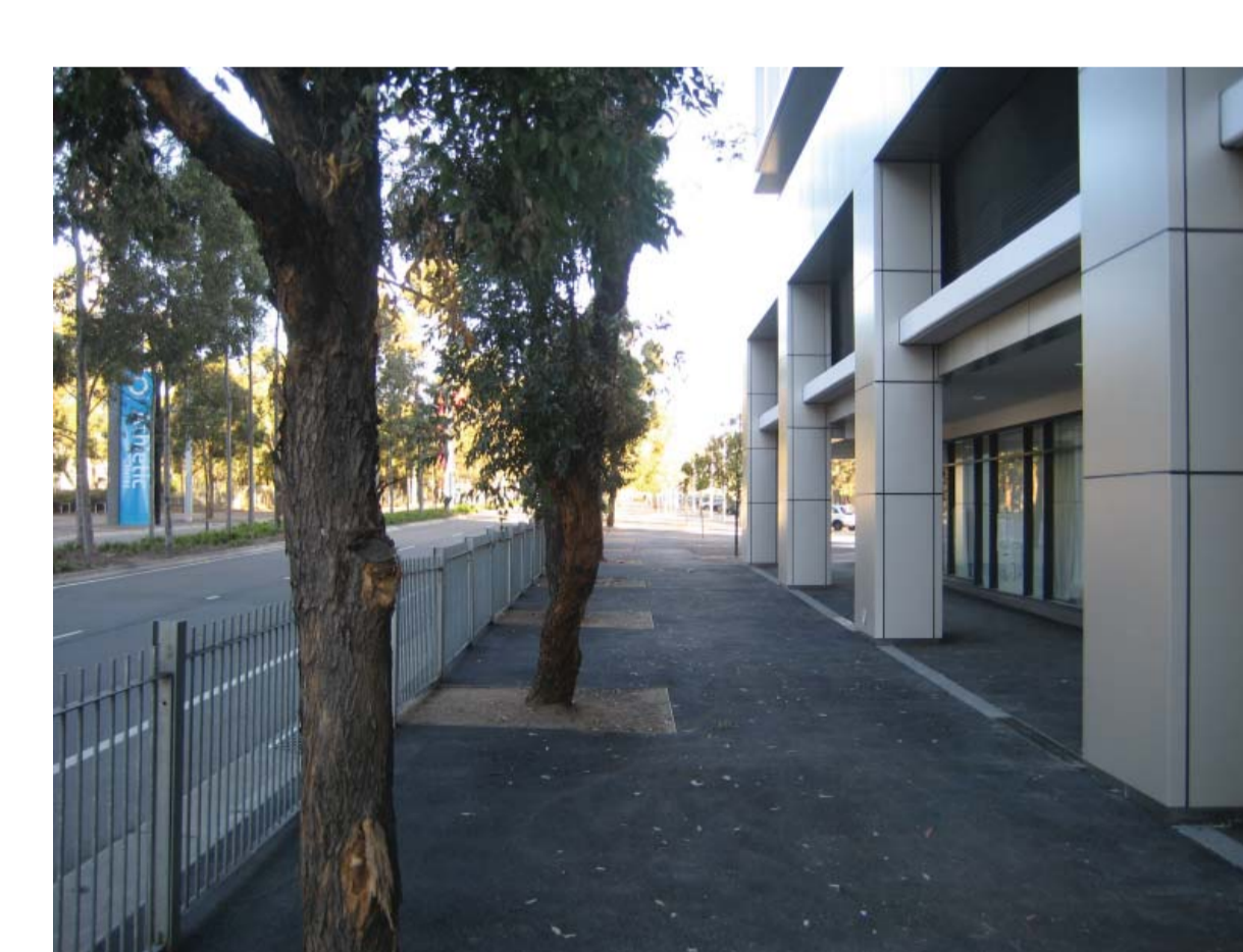
Existing Formula 1 hotel showing footpath width, and colonnade depth. These dimensions will be emulated on the Quest apartments site.
