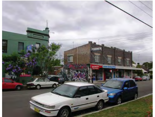
Figure 3.8 The northern boundary of the Struggletown Heritage Conservation Area from the opposite side of Barker Street. Note the mixed commercial nature of the place along this portion of Barker Street.
