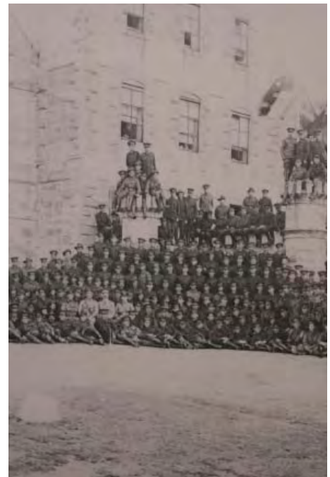
Figure 2.6 The Asylum was requisitioned by the federal authorities in late 1915 for use as a military hospital during the First World War. Source: Randwick, 1859-1976.
