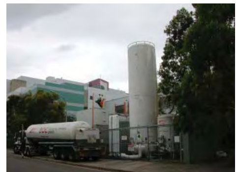
Figure 3.2 The western facade of Blackdog Institute seen from Hospital Road.
