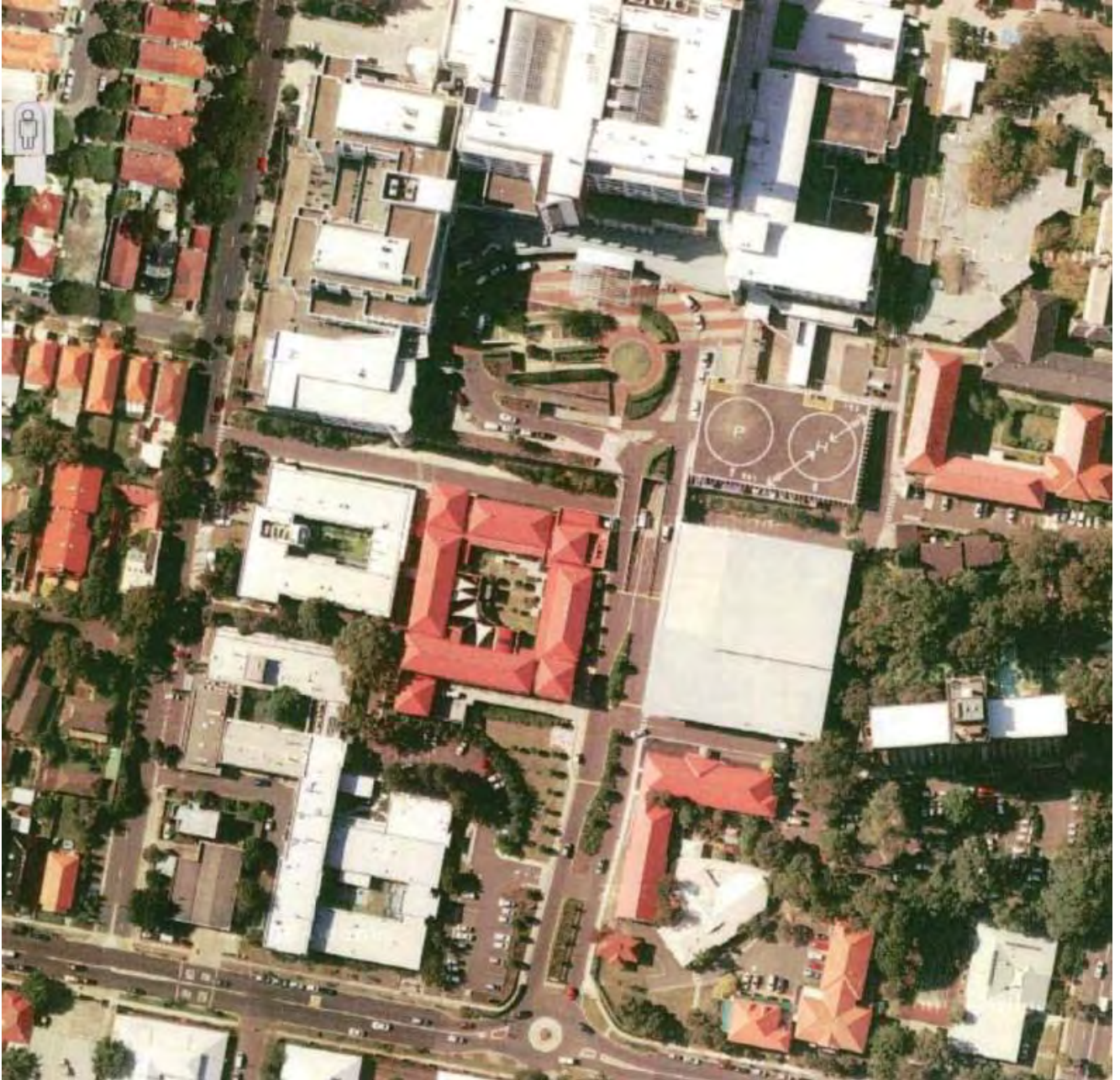
Figure 3.23 Current aerial photograph of the site. Source: Department of Lands
