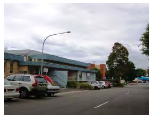
Figure 3.13 The rear of Villa 2 from Hospital Road.
