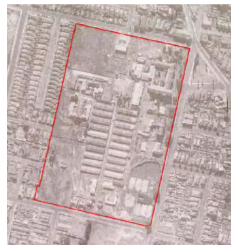
Figure 2.8 Aerial view of the Repatriation Hospital in 1943. Source: Department of Lands.
