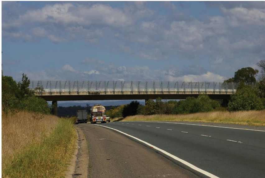
Fig. 6.17 Moreton Park Road Bridge (South)
