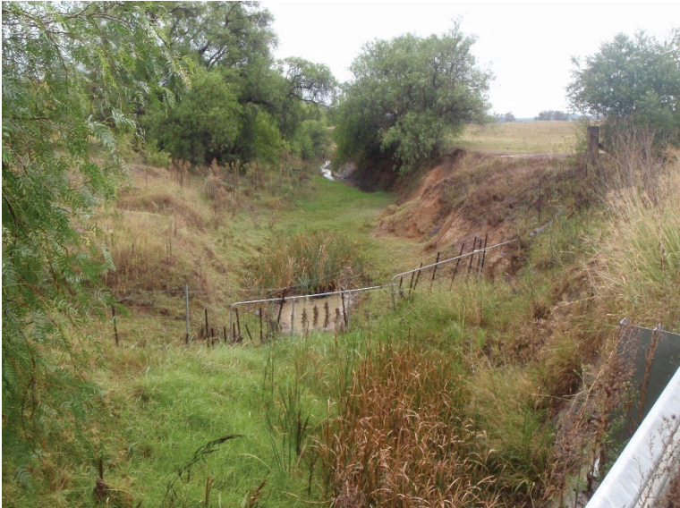
Fig. 5.1 Foot Onslow Creek (Source: IMC)
