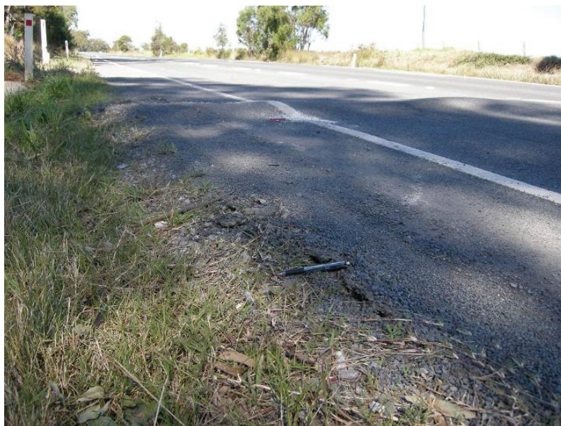
Fig. 6.7 Bump in slip lane along Appin Road above West Cliff Longwall 32 (Source: Colin Dove)
