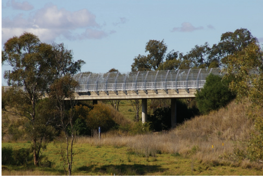
Fig. 6.16 Moreton Park Road Bridge (North)
