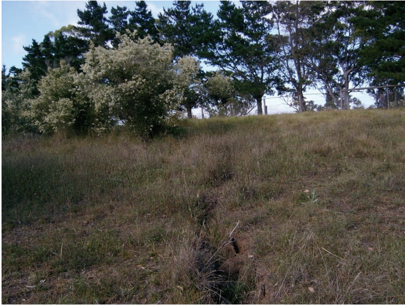
Fig. 5.18 Example of surface tension cracking along the top of a steep slope
