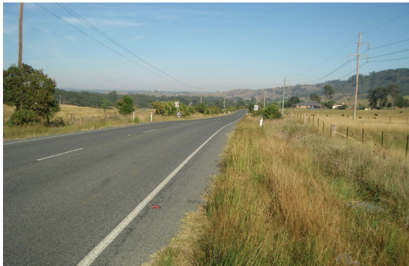
Fig. 6.20 66 kV and 11 kV powerlines along Menangle Road
