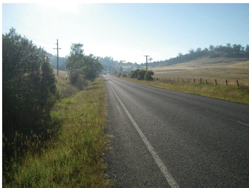
Fig. 6.6 Photograph of Menangle Road in Area 9
