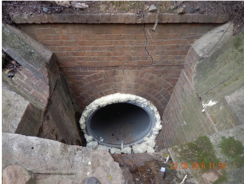
Fig. 6.4 Culvert at 69.0 km (prior to completion of mitigation works)
