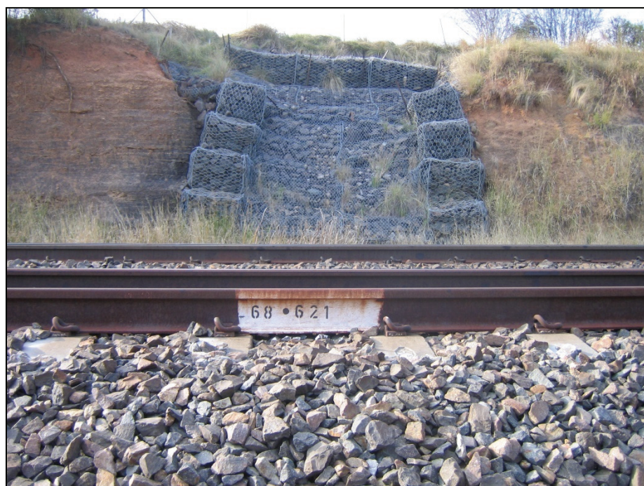
Fig. 6.2 Cutting at 68.6 km with gabion wall and race on down side
