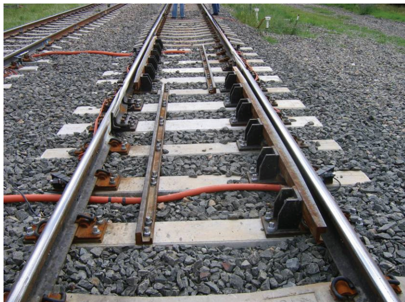
Fig. 6.5 Rail expansion switch
