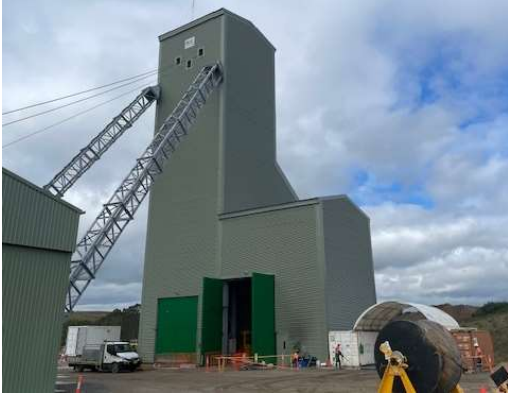
Plate 1: Acoustics designed VS8 Headframe building
