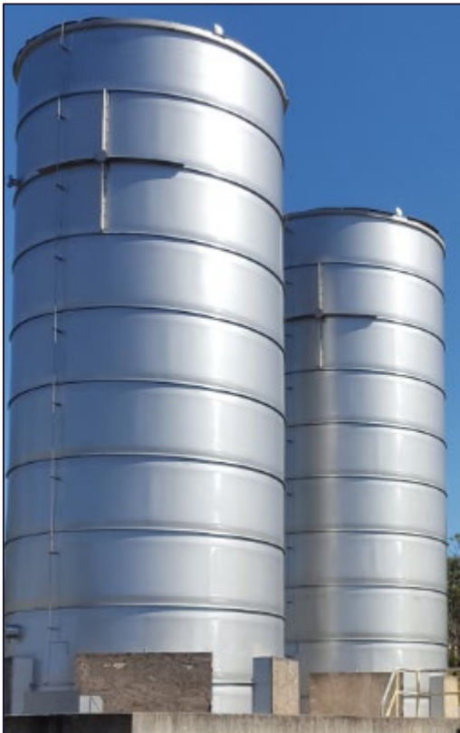
Plate 6: Vertical Flares (as used at permanent facilities)
