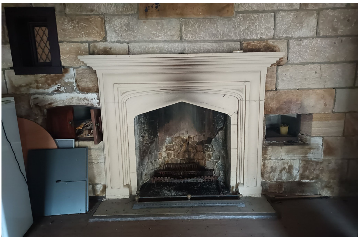
Plate 40. Replica York stone gothic revival fireplace surround and side ovens, now wood boxes. The inscribed 1865 panel can just be seen above (Source: Archive Heritage)
