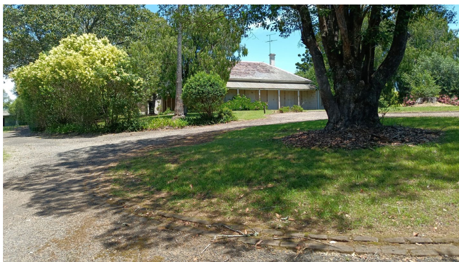
Plate 4. View west back toward the front verandah (Source: Archive Heritage)
