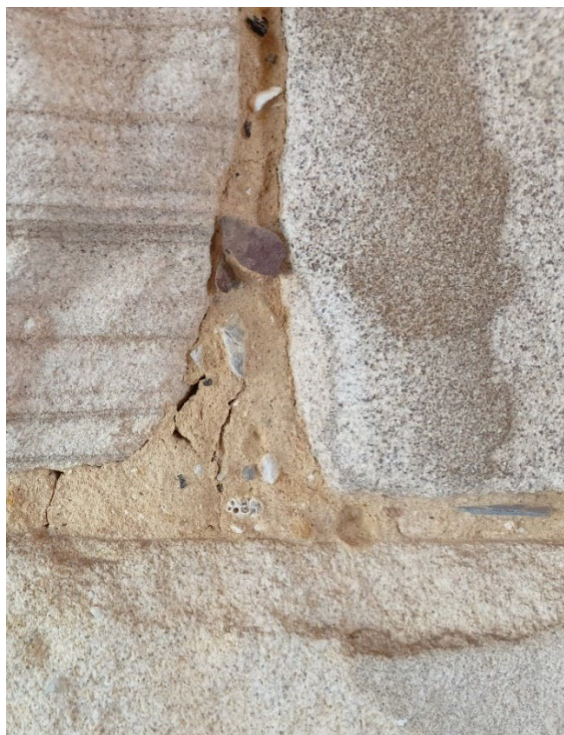
Plate 50. Detail of the mortar of the later stone masonry (Source: Archive Heritage)
