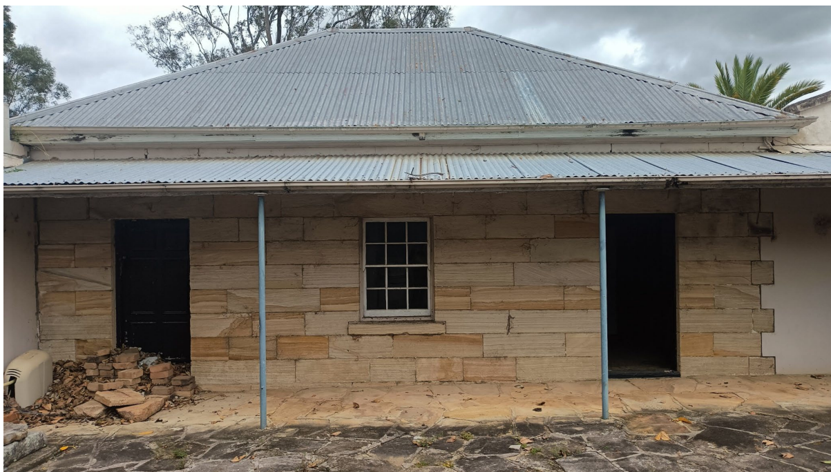
Plate 39. The symmetrical exterior (Courtyard) façade of the sandstone Kitchen (Source: Archive Heritage)
