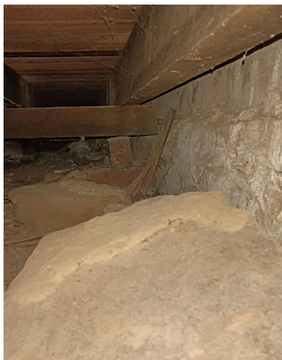
Plate 13. View of well-formed sandstone footings beneath interior floor (Source: Archive Heritage)
