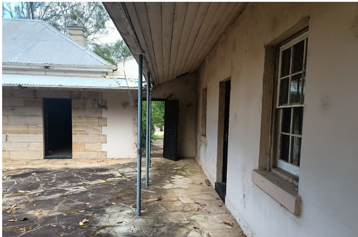
Plate 31. View west along front of the North Wing (Source: Archive Heritage)
