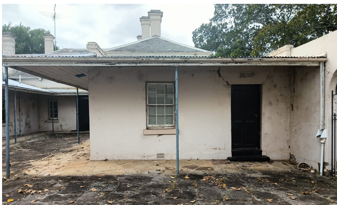
Plate 29. View east toward the later addition to the South Wing (Source: Archive Heritage)
