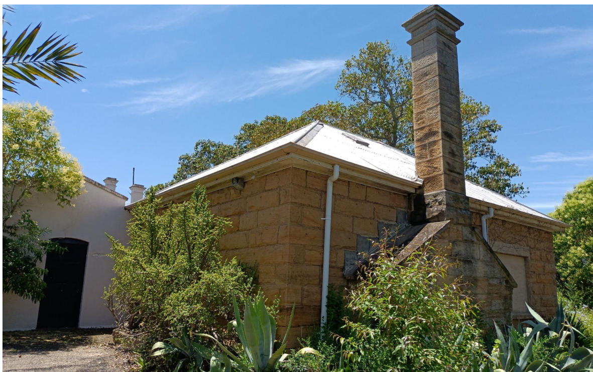
Plate 19. View south-east toward the western elevation of the Kitchen and attached Courtyard wall (Source: Archive Heritage)
