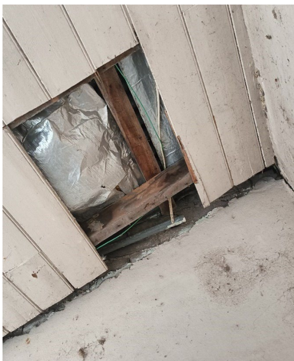
Plate 33. Timber board ceiling in Bedroom 4 (Source: Archive Heritage)
