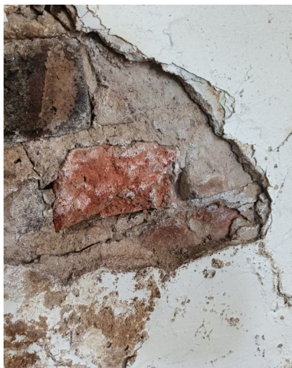
Plate 34. Early bricks and mortar beneath painted render in Bedroom 4. (Source: Archive Heritage)
