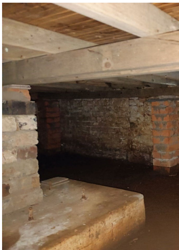
Plate 53. View north-west into the cellar showing large, central masonry base block with threaded iron fixing rods
