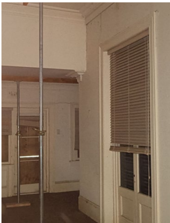
Plate 26. View north through the living room showing bulkhead of northern extension (Source: Archive Heritage)
