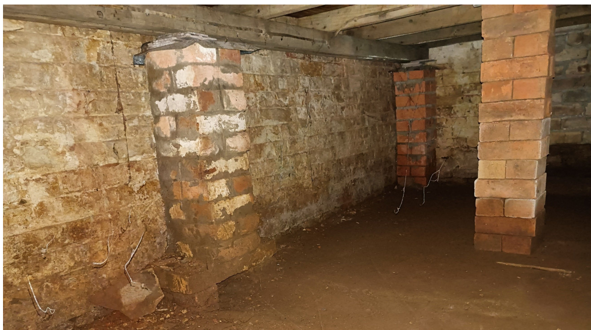
Plate 51. View south-west into the cellar subfloor area showing later brick piers supporting the Phase 3 floor (Source: Archive Heritage)
