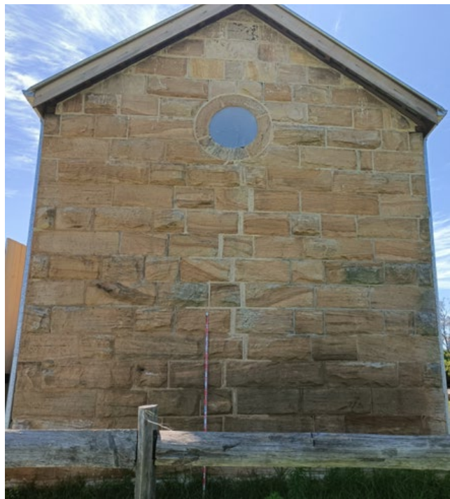
Plate 64. Current view of restored and conserved masonry and porthole (Source: Archive Heritage)
