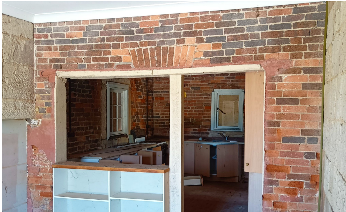
Plate 46. The splicing of the sandstone masonry into the brickwork can be seen at left (Source: Archive Heritage)
