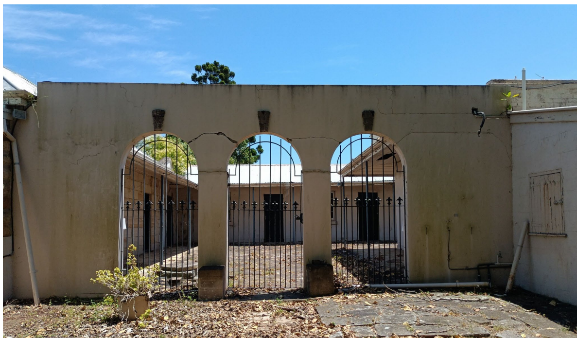
Plate 16. Phase 3 masonry arch wall exterior with the 20 th century laundry addition at right (Source: Archive Heritage)
