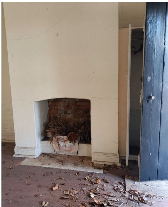
Plate 35. Original fireplace bricks in Bedroom 3
