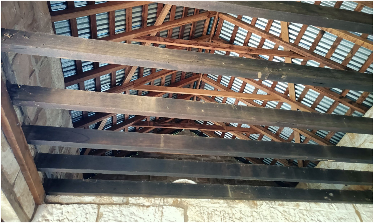
Plate 62. Restored roof over conserved loft floor joists as seen from Room 1 (Source Archive Heritage)
