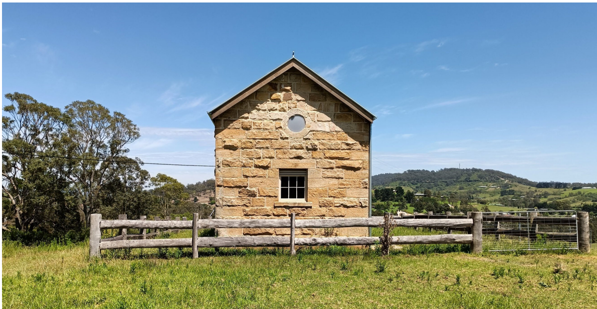
Plate 59. View west toward the Stable showing restored upper masonry and casement and porthole windows (Source: Archive Heritage)
