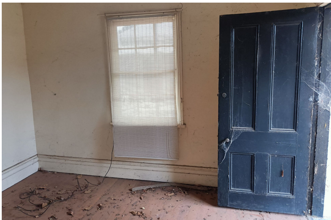
Plate 30. Interior of the Bedroom 5 western extension of the South Wing with original window (Source: Archive Heritage)
