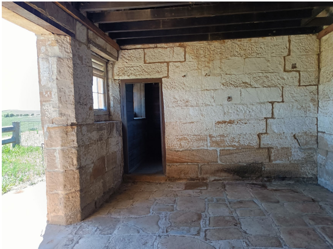
Plate 61. Interior of Room 1 showing restored stone walls and floor setts. Entry to the tack room (Room 2) is seen (Source: Archive Heritage)
