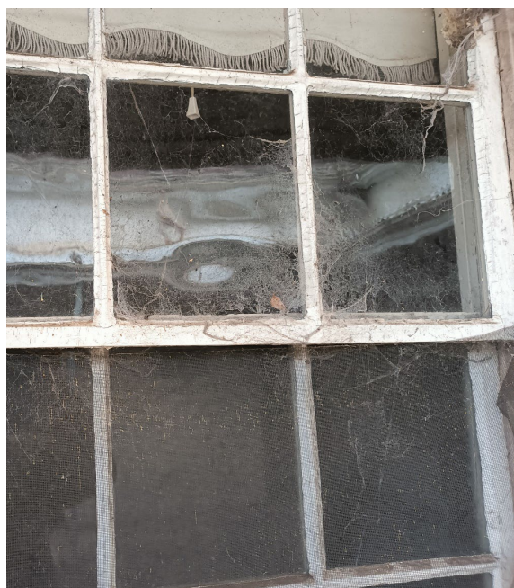
Plate 37. Warped, mid-19 th century cylinder glass in an original Bedroom 3 window (Source: Archive Heritage)
