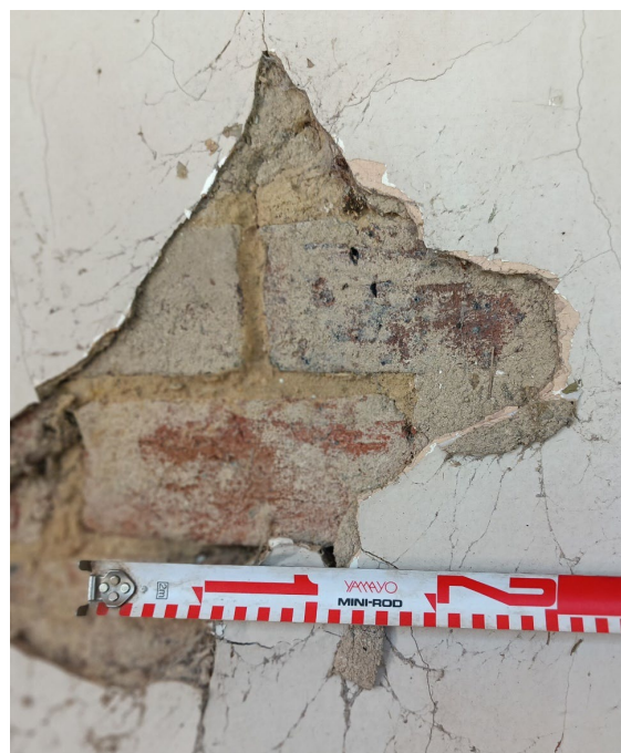
Plate 15. Detail of render and mortar (Source: Archive Heritage)
