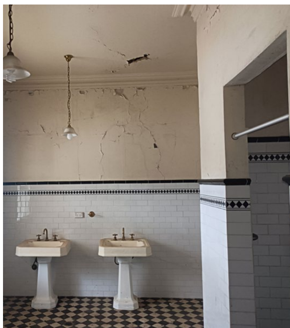
Plate 38. Phase 3 Bathroom 2 (Source: Archive Heritage).
