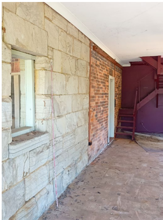
Plate 57. Interior view of the former exterior junction of brick and sandstone and the 20 th century addition with first floor stairs in background (Source: Archive Heritage)
