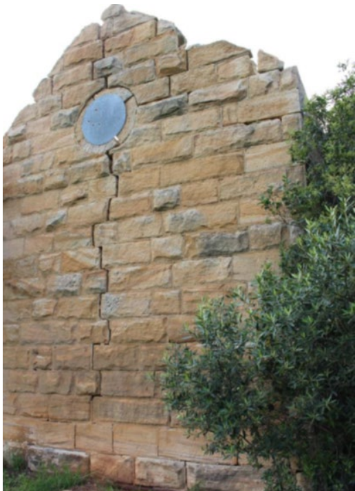
Plate 63. Western elevation as seen prior to restoration works in 2021 (Source: Niche 2019: p.14)
