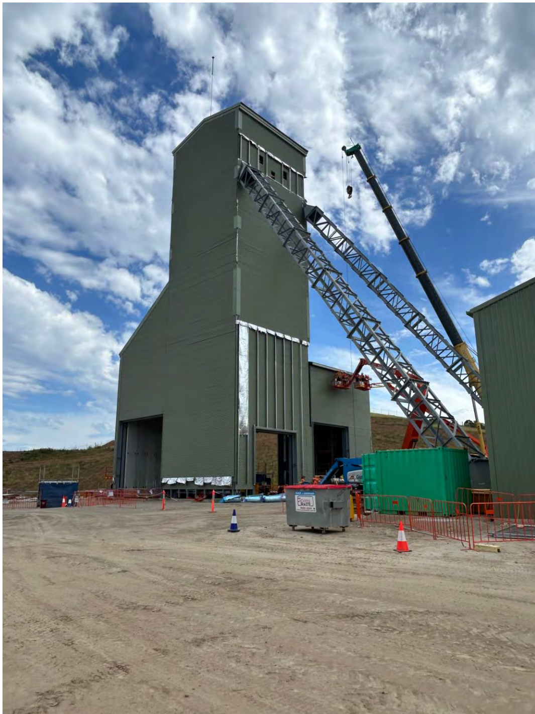
Figure 3. Headframe Currently Under Construction
