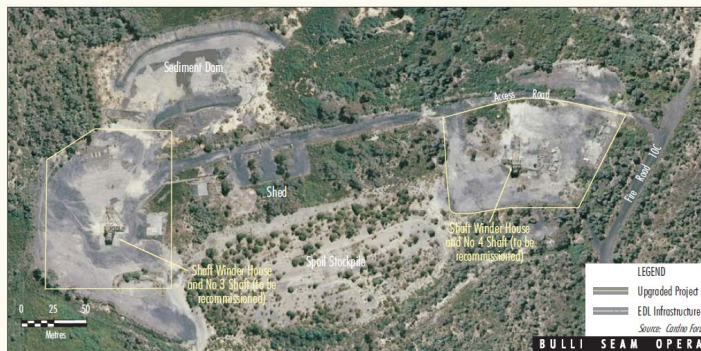
North Cliff Shafts
