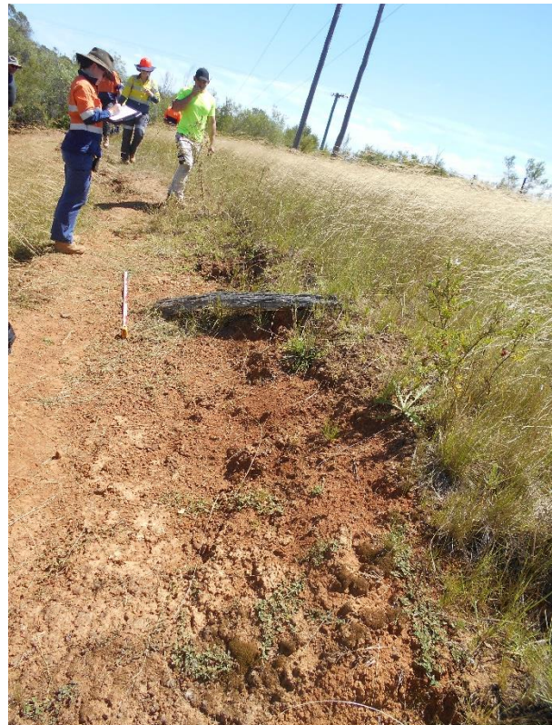
Plate 19: Bulli Site 8 (AHIMS ID#52-2-3688) area of eroding exposure along fence line. Facing north.
