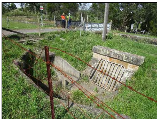
Plate 3: Sandstone culvert and discharge channel running beneath the Upper Canal on the north side of Brooks Point Road, looking south west.
