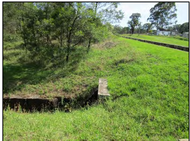
Plate 12: Sandstone discharge channel running west beneath the Upper Canal on the north side of Brooks Point Road, looking north.
