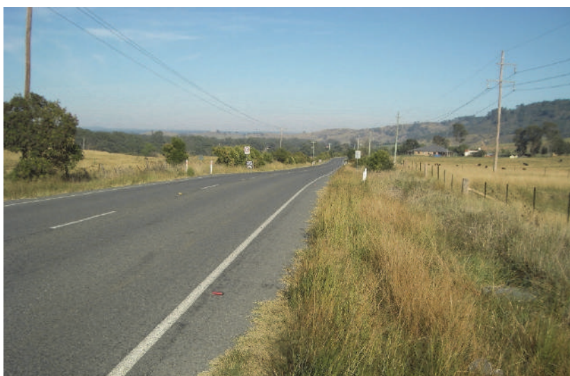
Fig. 6.9 66 kV and 11 kV powerlines along Menangle Road
