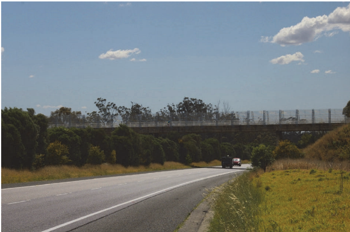
Fig. 6.6 Moreton Park Road Bridge (North)
