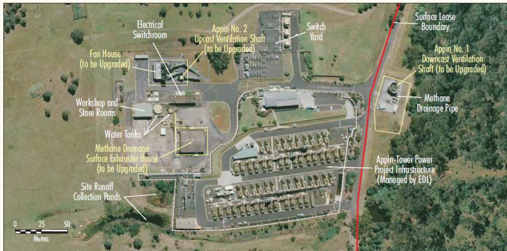
Appin No 1 and No 2 Shafts
