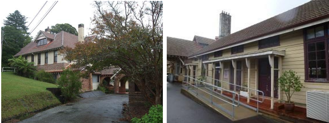
Figure 5 Aged Care Building Structure Refs. B02a and B02b
