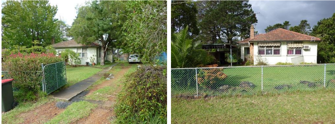
Figure 7 Houses Structure Refs. B06a (left side) and B08a (right side)
