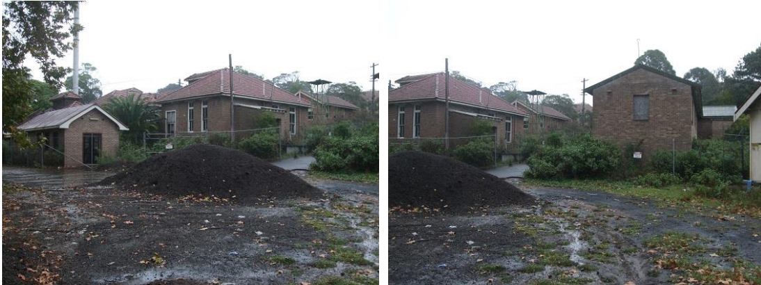
Figure 2 Hospital Building Structure (Ref. B03a)
