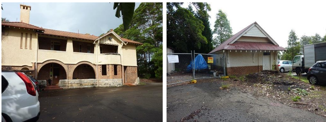
Figure 6 House Structure Ref. A09a (left side) and A09b (right side)
