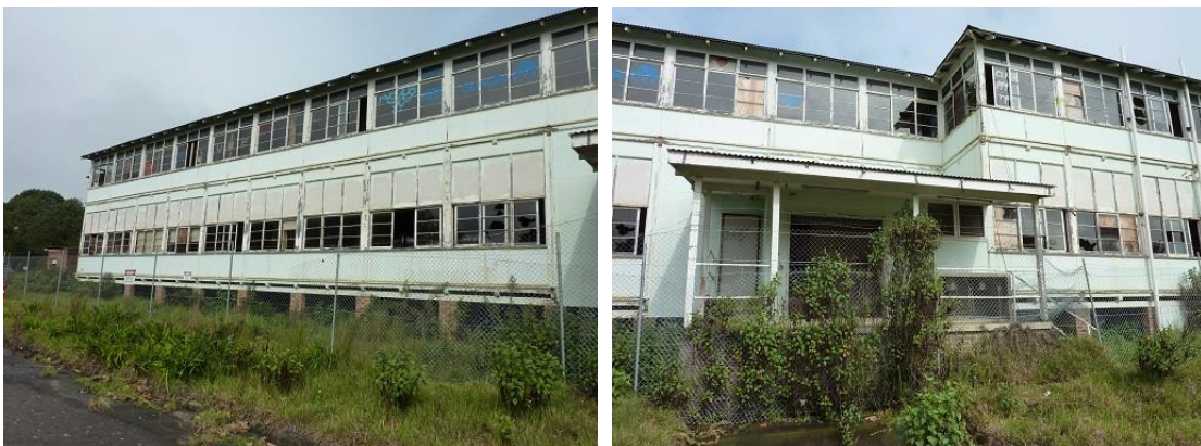
Figure 1 Hospital Building Structure (Ref. A01a)
