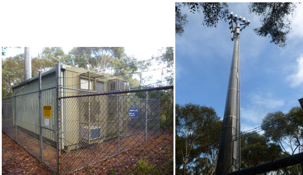
Figure 1 Telecommunications Tower and Compound
