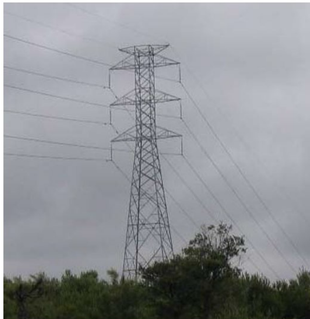
Plate 1 – 132 kV Transmission Tower (Source: MSEC, 2016)
