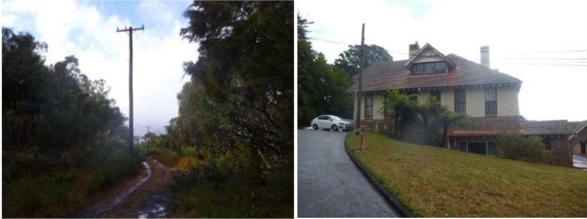
Plates 2 and 3 – Aerial Powerlines (Source: MSEC, 2016)
