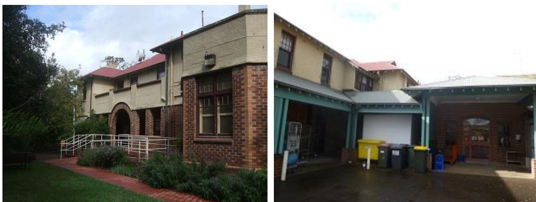
Figure 4 Aged Care Building Structure Ref. B01e
