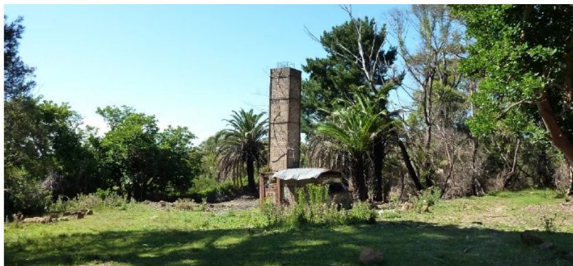
Plate 20 – Kiln (Source: JMA, 2016)
