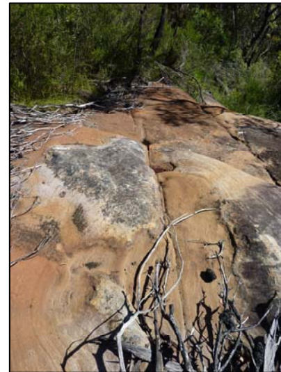
TB069-5 Joint with water
