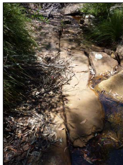
TA23-3 Joint downstream of Pool TA-I
