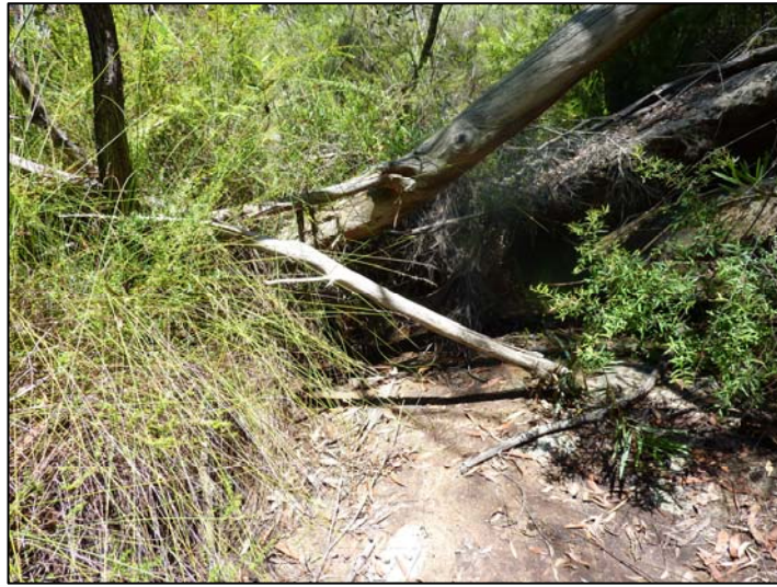
TA18-1 Upstream end of rockbar looking Upstream
