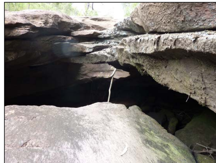
TB146-4 Pothole in overhang
