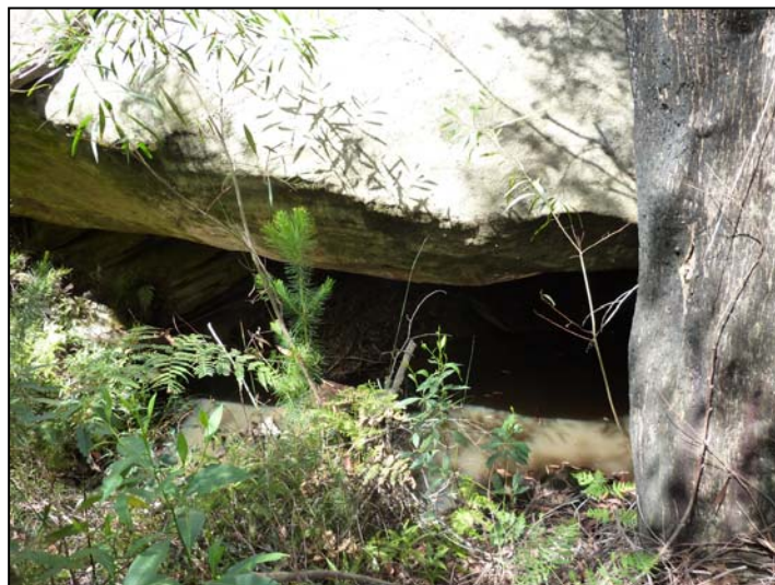
TB100-5 Overhang on southern bank
