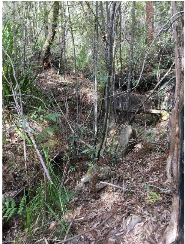
Photo S1 (Upstream)
