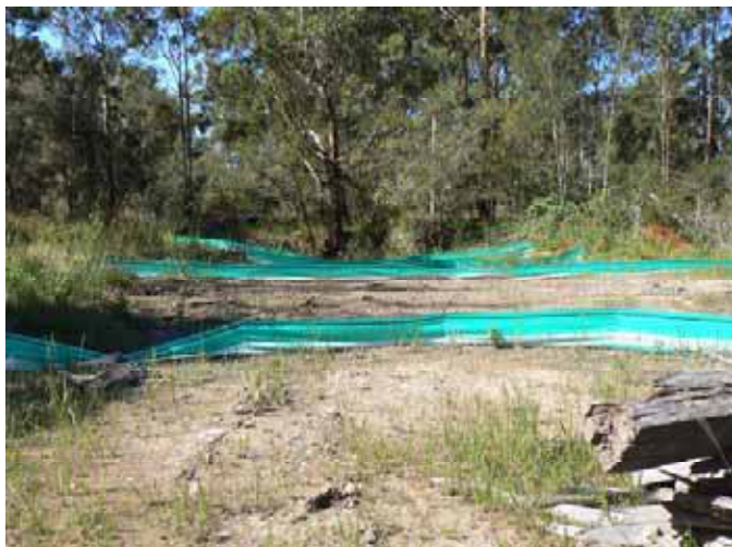
Plate 9: Silt fences protect Double Crossing Creek , 2009
