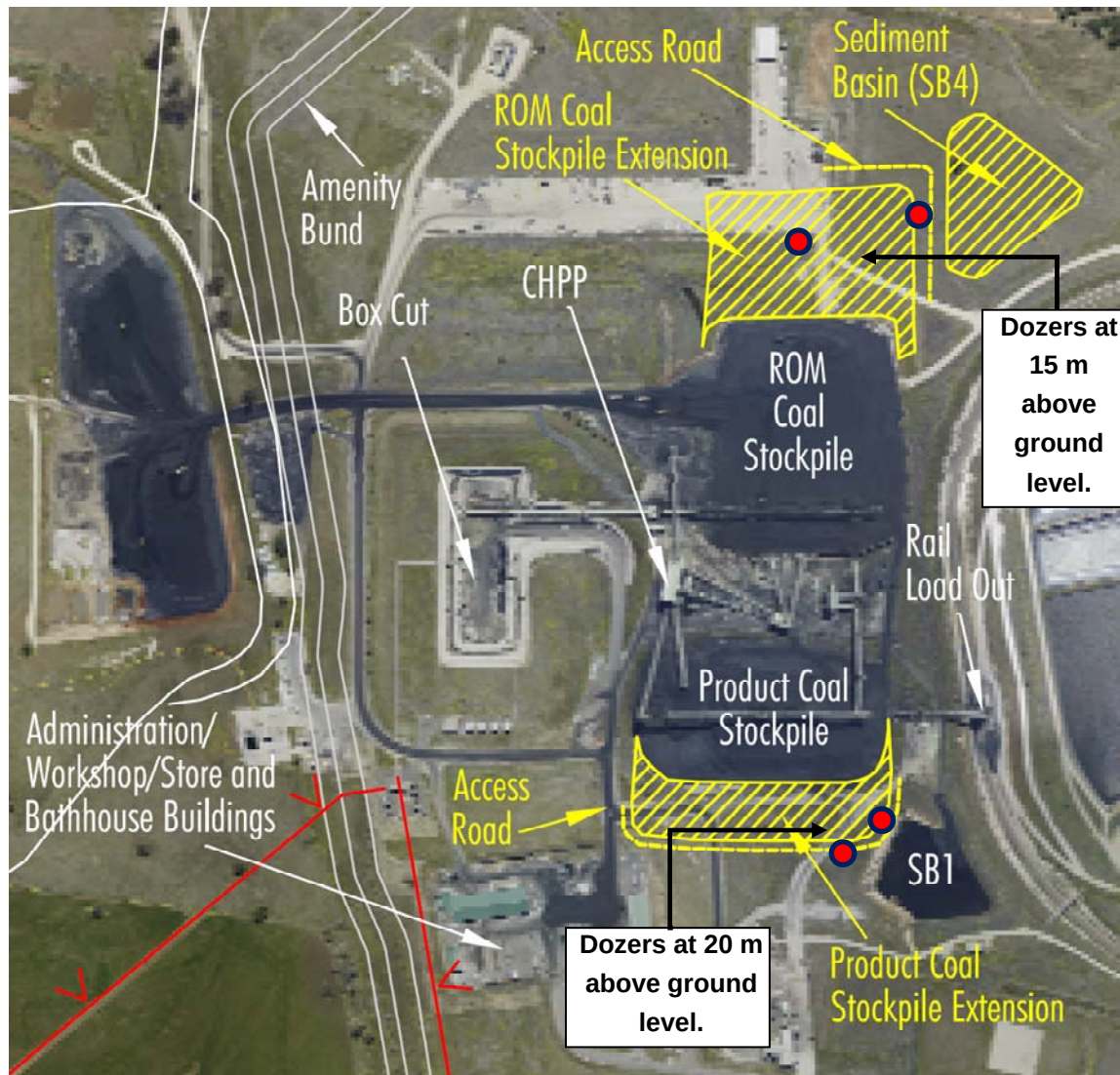
Figure 3. ROM and product coal stockpiles expansion.
