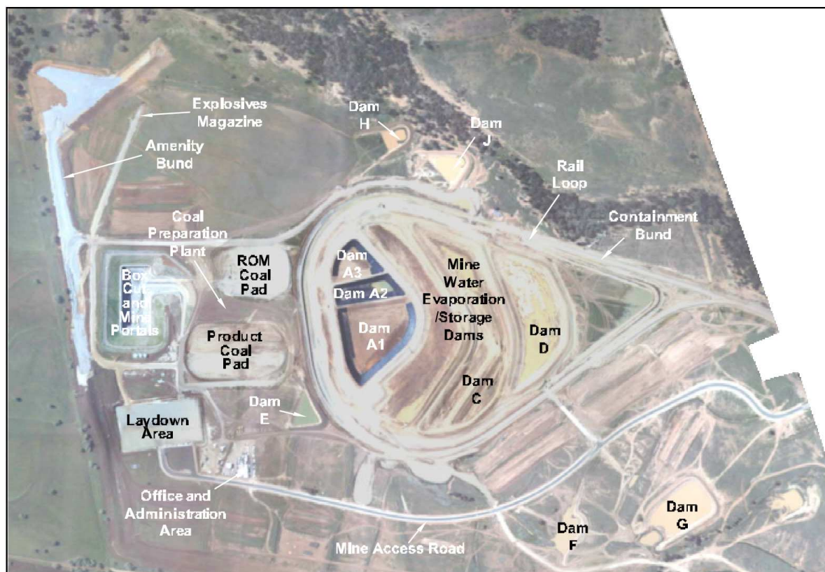
Figure 3: Aerial View of Stage 1 Pit Top (under construction 2009)
