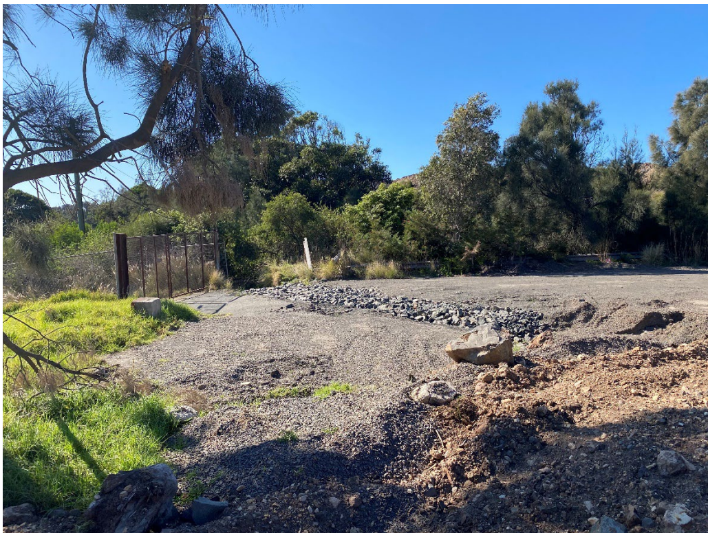
Photo 14: Temporary ESC measures in place along eastern side of site near the emergency access gate.
