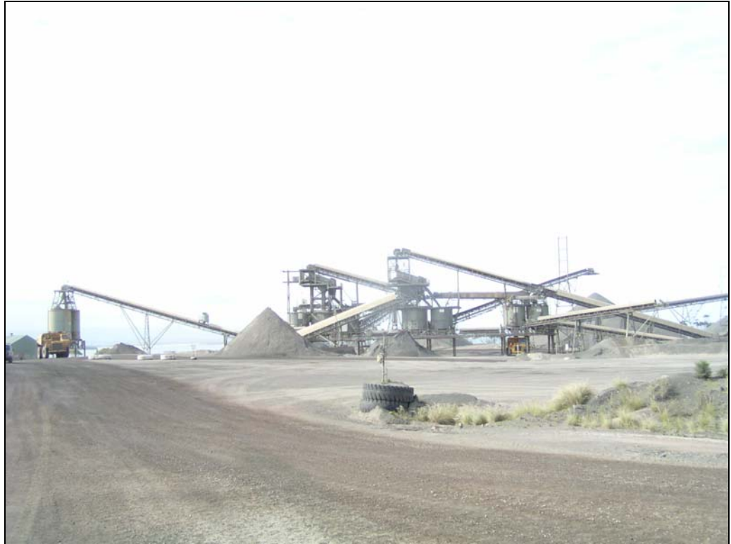
Figure 2: Photograph of the existing processing plant area to be rehabilitated and used for effluent disposal (24/11/2009).
