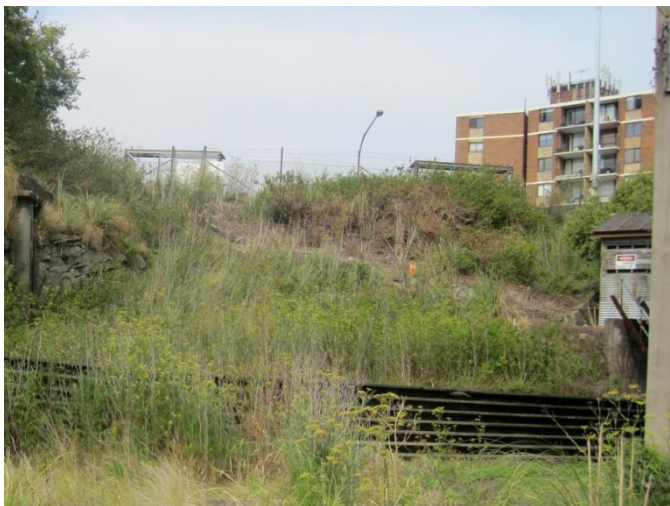
Figure 2-3 Location of the proposed widened share path in the White Bay Power Station. This area is the embankment immediately behind the existing bus stop. The construction of a retaining wall is not required.
