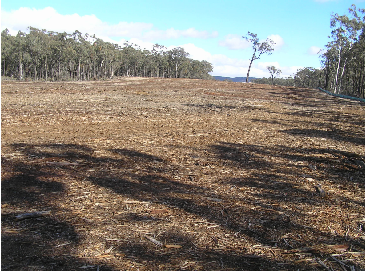
Plate 1. Stage 1. Mulched timber has been left insitu and will be mixed with topsoil during the topsoil stripping process.
