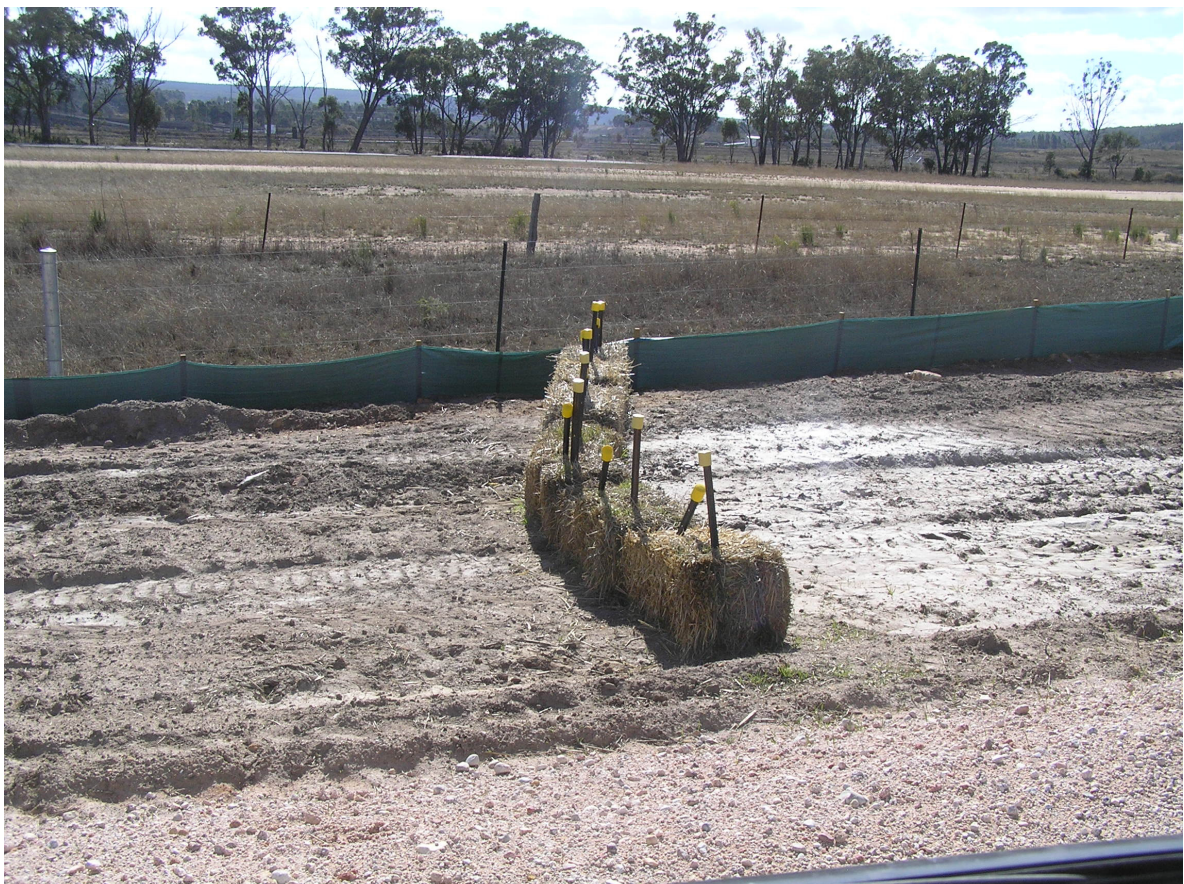
Plate 6. Stage 1. General erosion control structures appear adequate.
