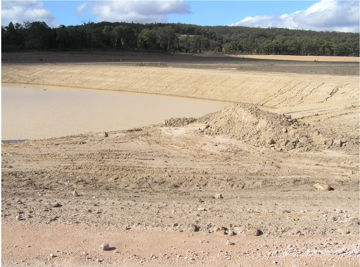
Plate 3. Stage 1. Surface water management structures appear to be well designed and constructed.
