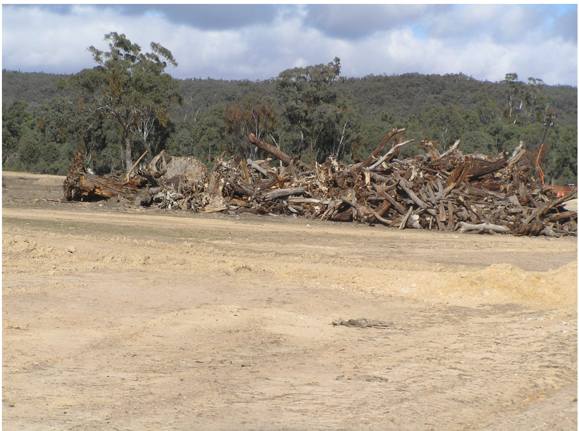
Plate 2. Stage 1. Timber considered too large for mulching has been stockpiled and will be deposited onto rehabilitated areas.
