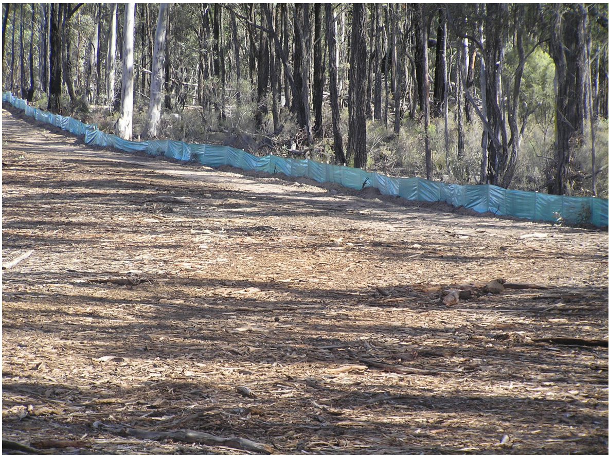
Plate 4. Stage 1. Approximately 50 km of sediment control fencing has been installed. Good techniques appear to have been employed.
