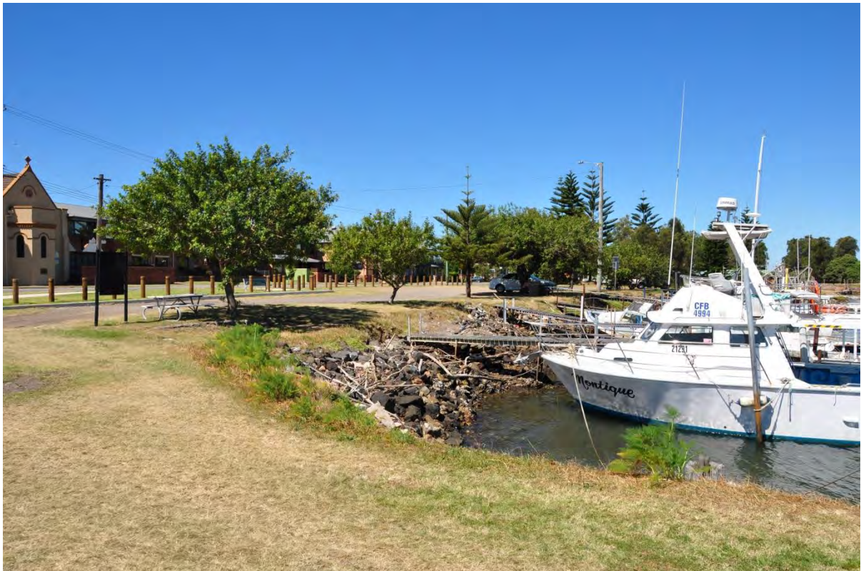
Plate 4 Typical foreshore treatments near S2
