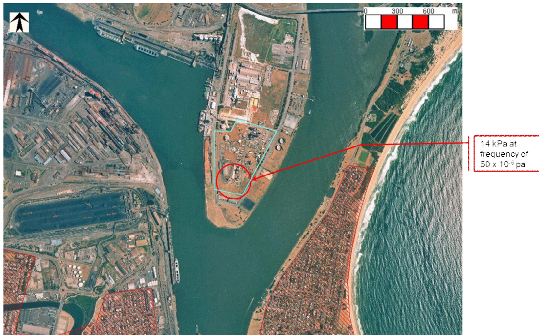
Figure 3-12: 14 kPa Overpressure Explosion Property Damage and Propagation Risk – PHA
