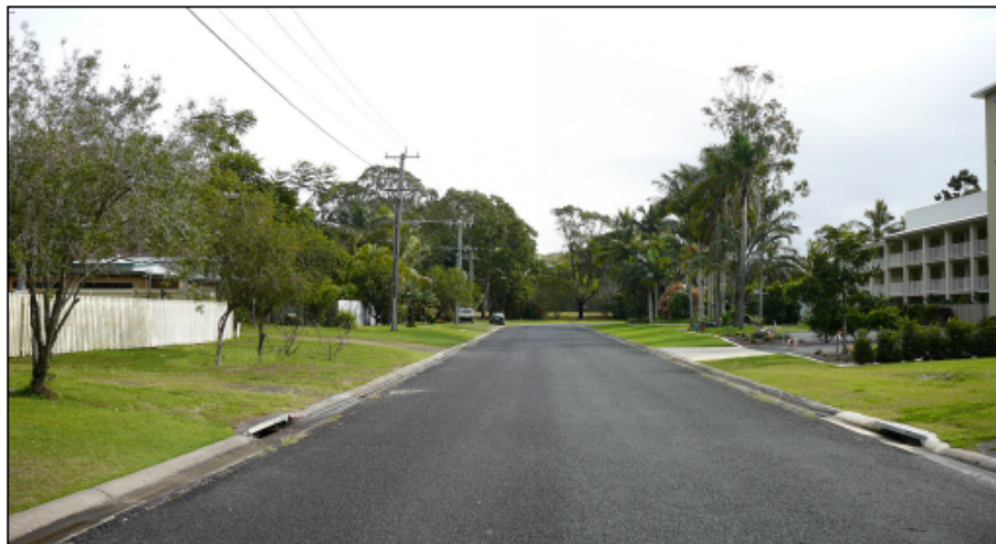
Figure 12: View to site from Tamarind Avenue.
