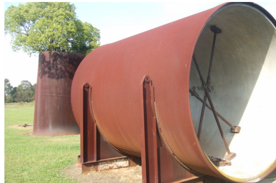
Defunct water carrier pipes with structural re-enforcement
