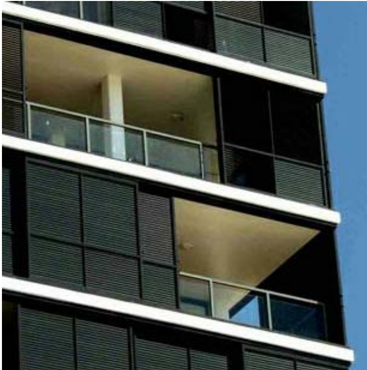
Prefinished Metal Framed Sun Screen Panels To Residential Levels
