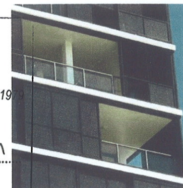
Finished Metal Framed Sun Screen Panels To Residential Levels
