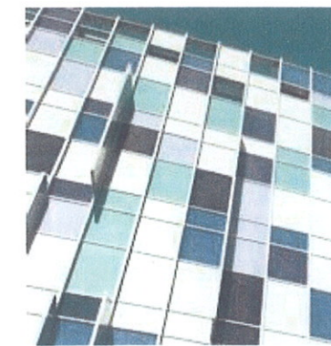
Finished Aluminium Framed Feature Screen
