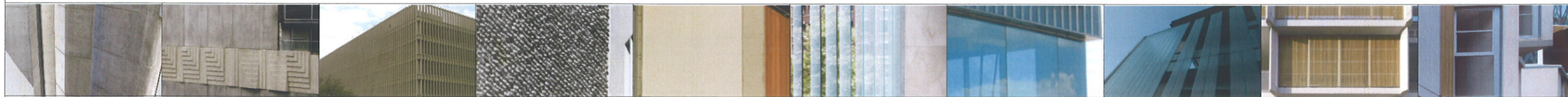
(A) OFF FORM CONCRETE (B) PRECAST CONCRETE (C) PRECAST CONCRETE SCREEN (D) PROFILED PRECAST CONCRETE (E) PAINTED CONCRETE (F) GLASS FINNS (G) SHOPFRONT GLAZING (H) U PROFILE GLASS SCREEN (L) TIMBER SCREEN (M) ALUMINIUM FRAMED WINDOWS
